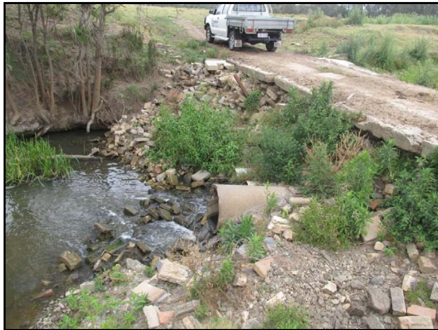
Photo 4: Close-up of the bridge, showing its construction from refractory brick.
